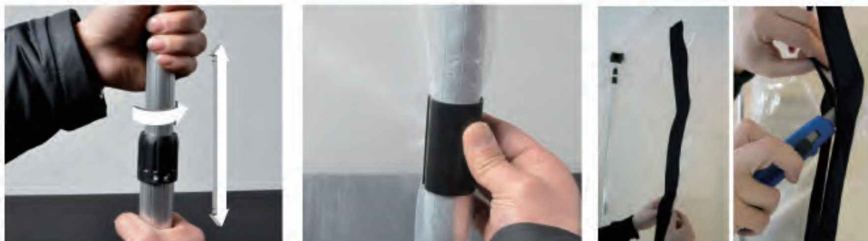
4. Adjust the pole length and lock into position with clock-wise twist. 5. Secure the sheet vertically with the U-clips. 6. To create an access: apply the adhesive zipper, open and cut the sheet following the zipper.
